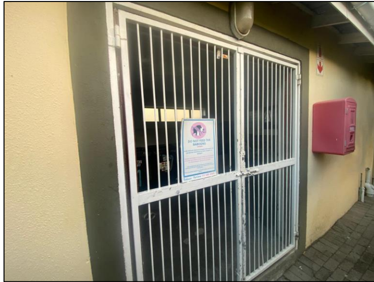
Figure 6. The secure waste room at Glen Mews.
